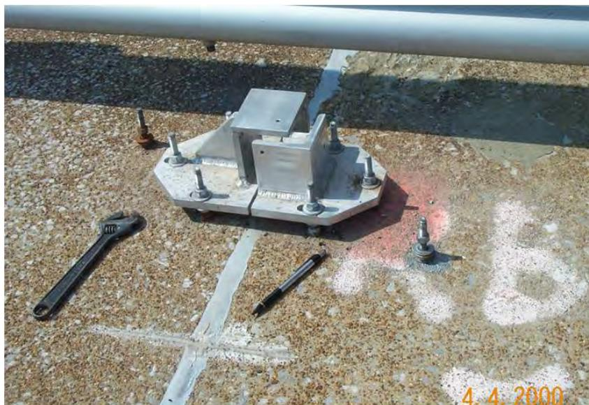
Relative movement device for three directions on a concrete joint requires precision installation
