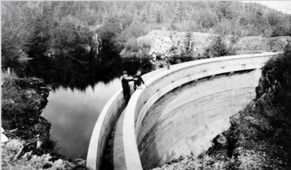
5 th Street Douglas Dam
