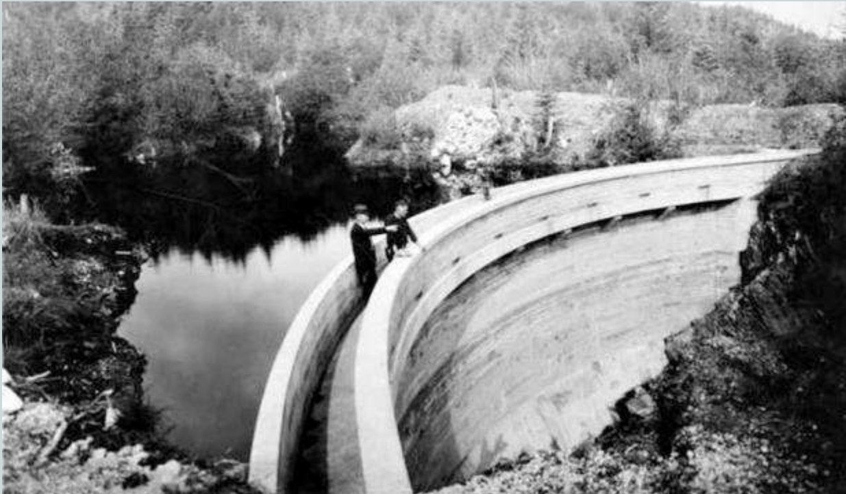
5 th Street Douglas Dam
